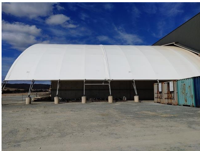
CONCENTRATE LOADING DOME CANOPY
