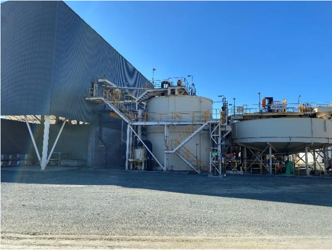
CONCENTRATION THICKENING AND FILTRATION
